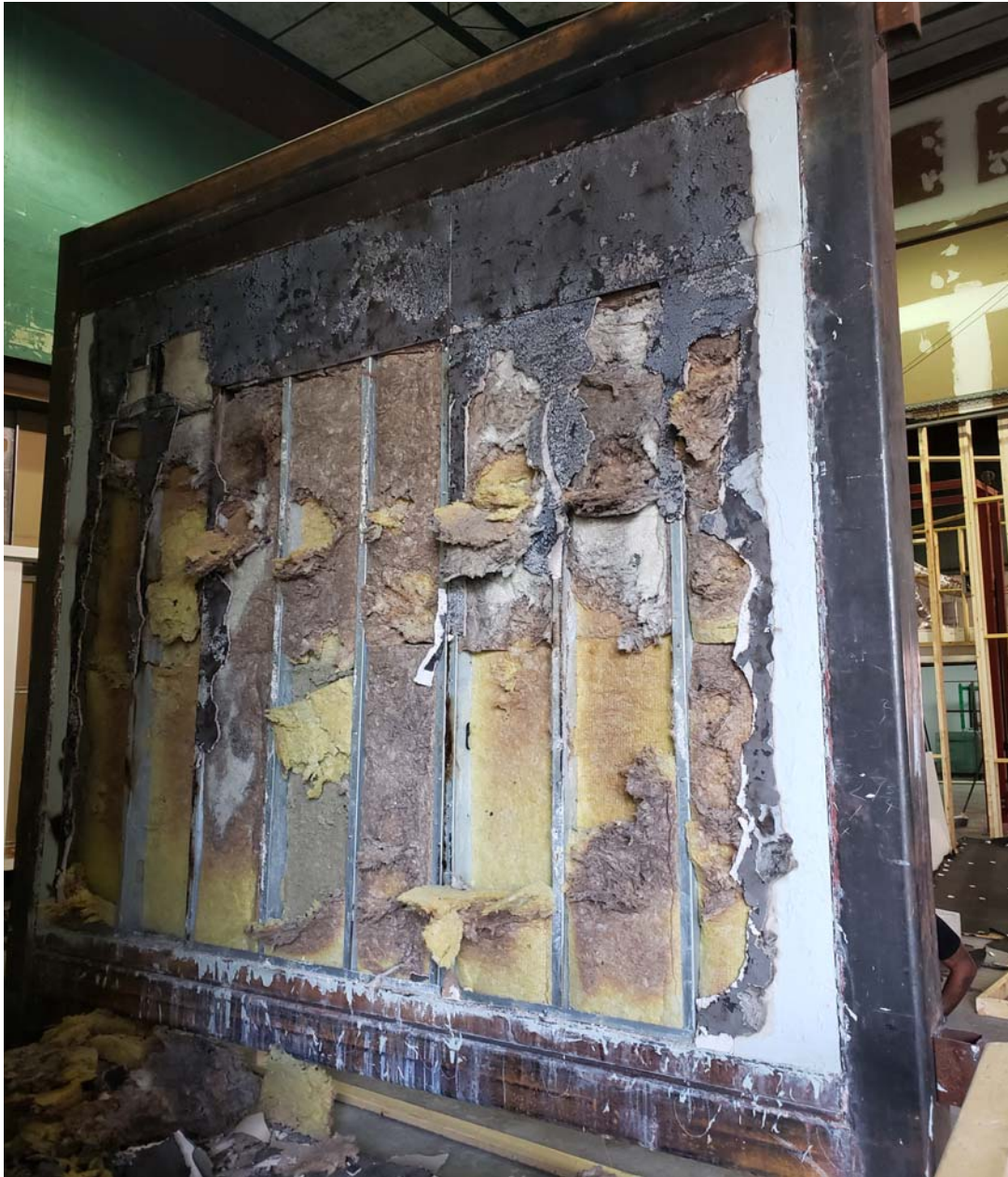
Figure 9: The exposed face of wall assembly after the hose stream test.
